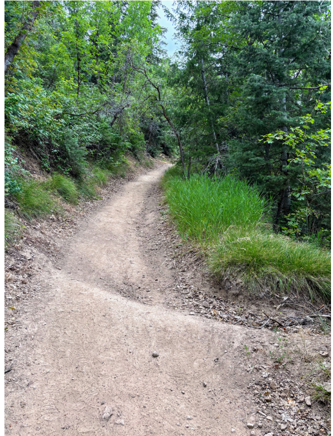
Water bars across the Switchbacks are necessary to push water off the trail.
